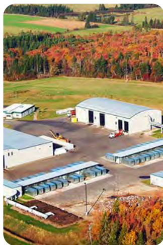
Central Compost Facility
