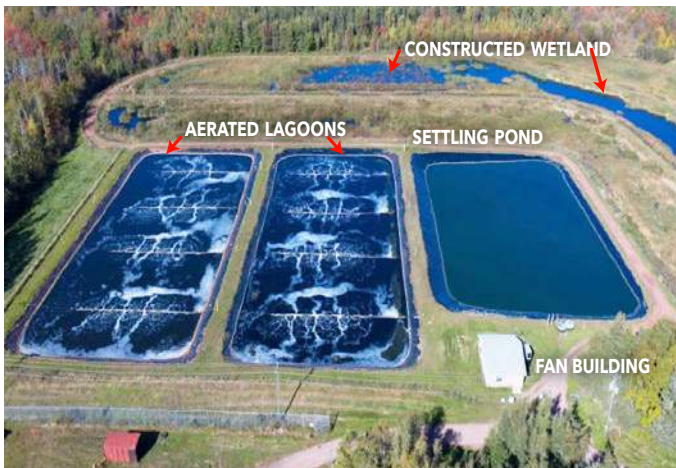
LEACHATE TREATMENT SYSTEM, EPWMF - October 2021
